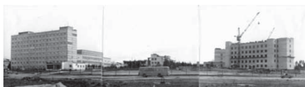
Рис. 8. Строительство Медгородка, 1987 г. Fig. 8. Building of healthcare city, 1987
